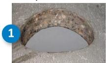
Drilling of hole with a diamond drill, upright to the pipe Drill hole  $\emptyset$  200 mm +/- 1 mm. Cleaning of the borehole.
