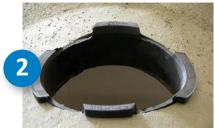
Position the rubber sealing ring in the drilled hole with the small and inscribed brace in the direction of current. Push the brace firmly into the pipe. Do not use any grease or lubricant when installing the sealing ring.
