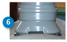
Take care the rubber braces/tabs will be placed between the notches of the connector and will be visible after assembly. Push in the PVC connector till it rests on the concrete pipe.
