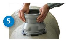
Position the PVC connector centric in the rubber sealing ring. Please note that the notch in the PVC connector points in the direction of current.
